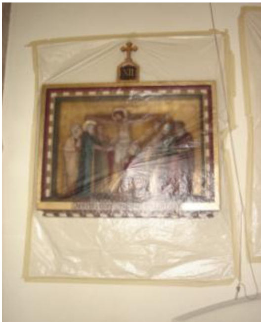
Protection for trial pit investigation only – bespoke timber casings were used for the main project
