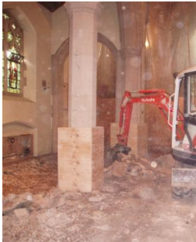
Protection for trial pit investigation only – bespoke timber casings were used for the main project
